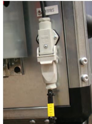
A typical quick-fit connection for a damper motor.
